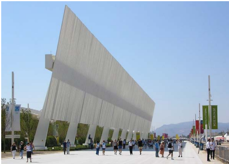
Figure 5: The Wall of Nations designed by S. Calatrava, Athens Olympic Sports Complex (Photo by the author)
